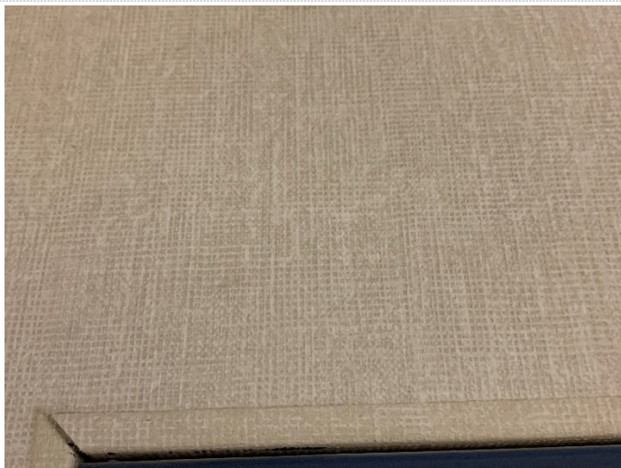
Tackboard and Glue on Drywall
